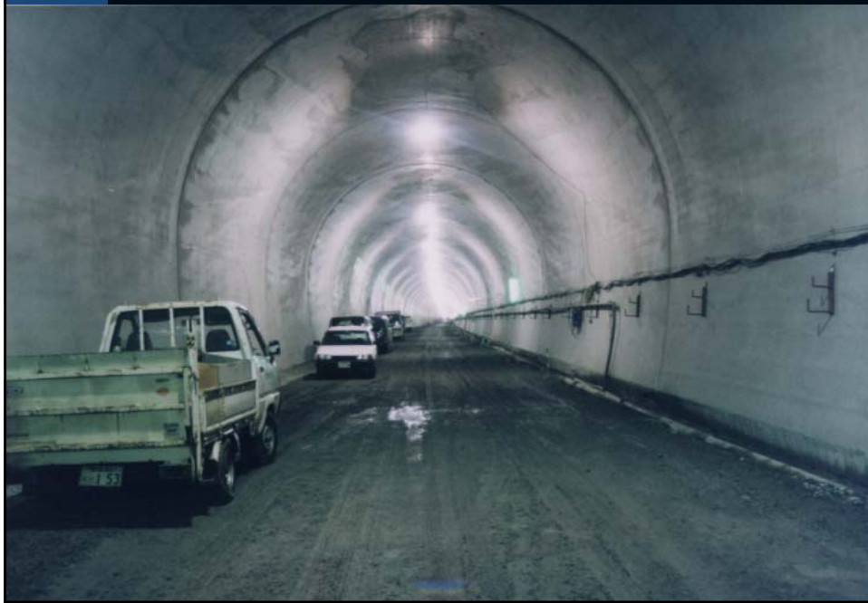
Interior view of the tunnel after placement of inner lining
